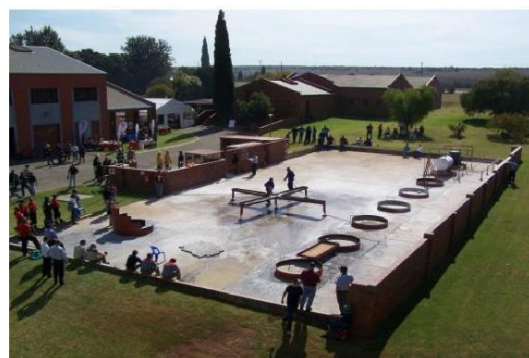
Large outdoor practical fire facility
