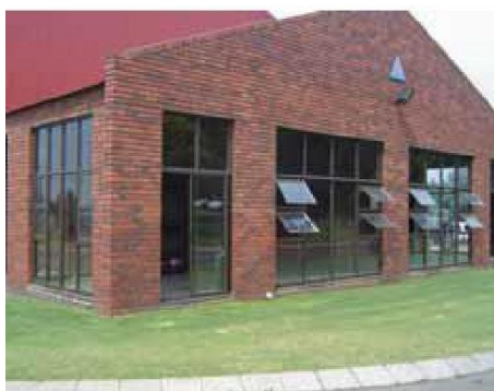
Fire House with technical workshops & live indoor fire facility
